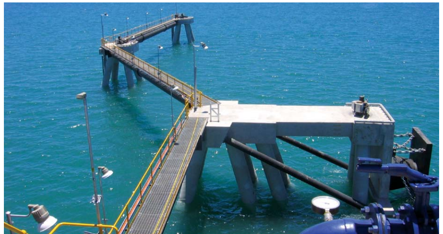
Walkway; Dampier Bulk liquids berth, Western Australia
