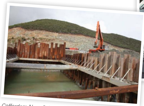
Cofferdam New Caledonia
