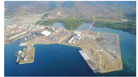
Motukea Bulk Cargo Wharf and Container Terminal, PNG
