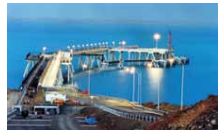
Dampier Bulk Liquids Berth, Western Australia
