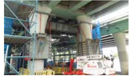
Riverside Expressway Bearing Replacement, Brisbane
