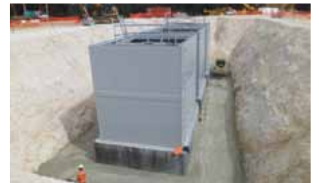
Gas Wellhead Foundations and Cellars, Southern Highlands, PNG
