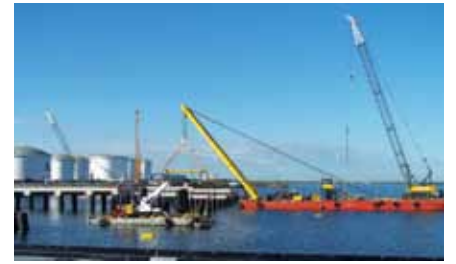
Barge Shear Leg, New South Wales
