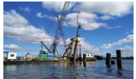
Barge Mounted Piling Frame, Brisbane
